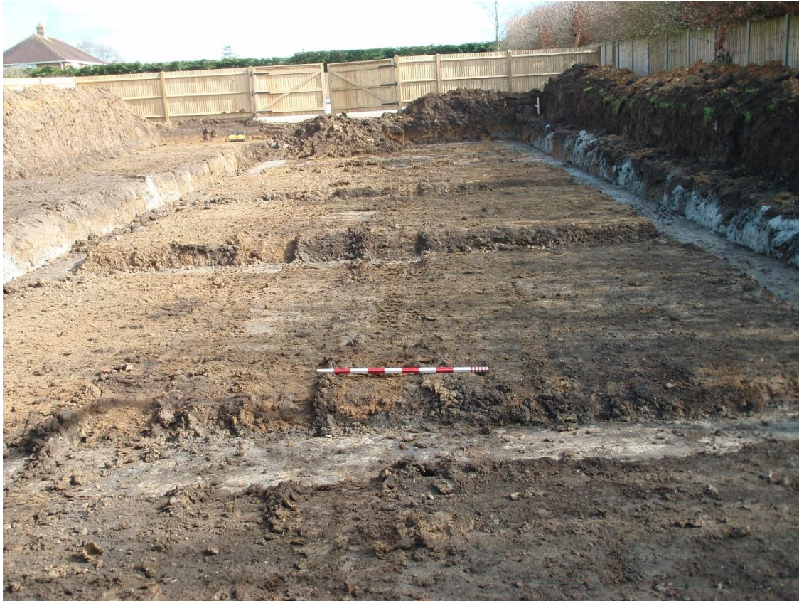
Plate 7. Subsoil strip completed and strip foundations completed
