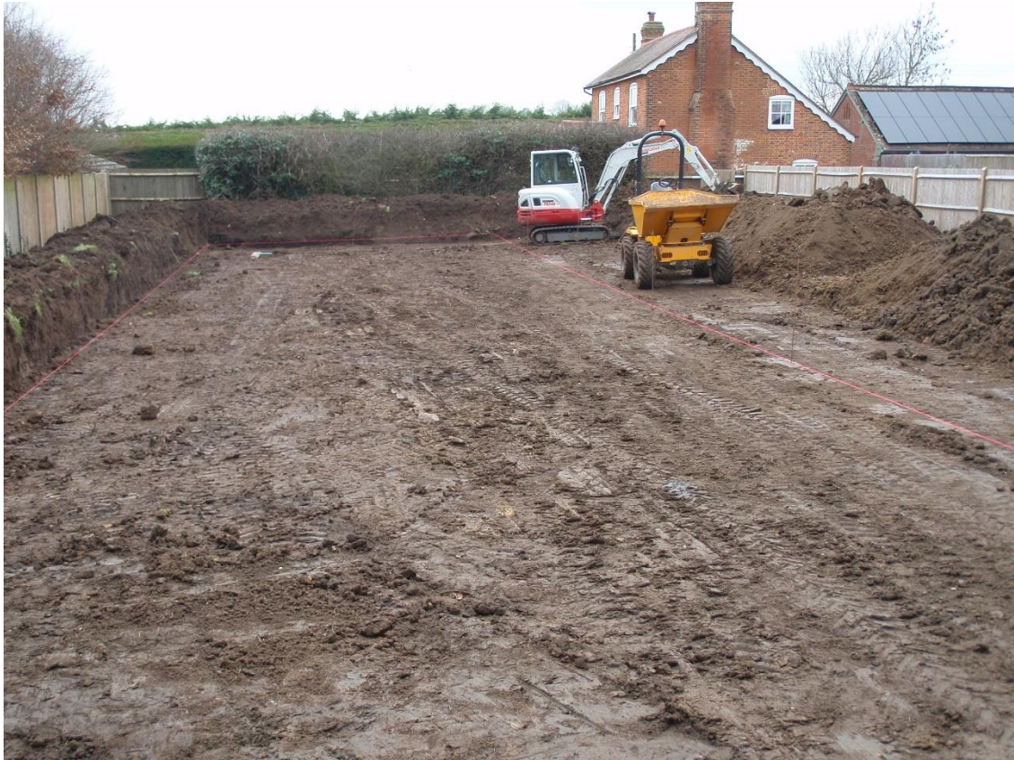
Plate 3. Topsoil/subsoil strip completed (looking west)
