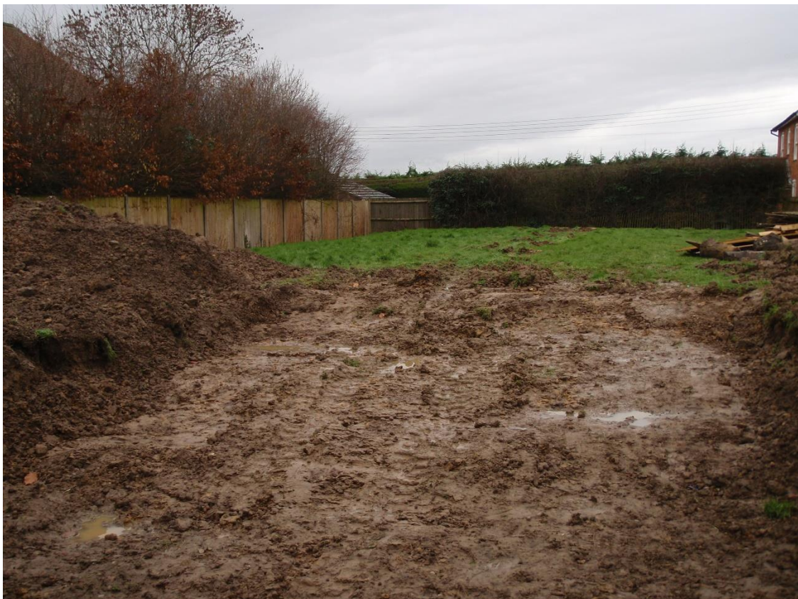
Plate 2. Topsoil strip (looking east)
