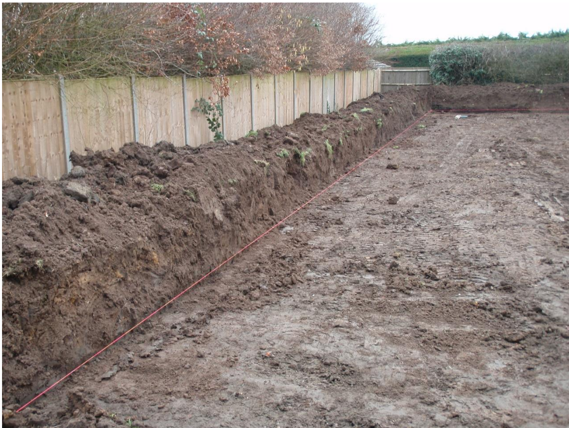
Plate 4. Topsoil/subsoil strip completed (looking SE)
