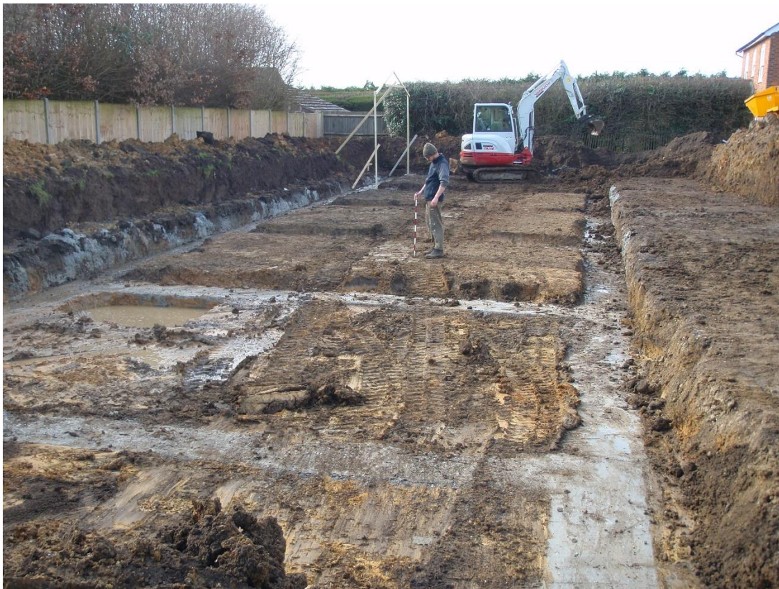
Plate 8. Completing east end subsoil strip
